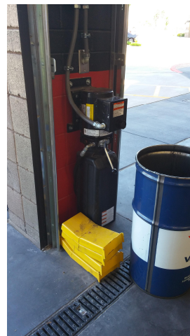
230v power unit
